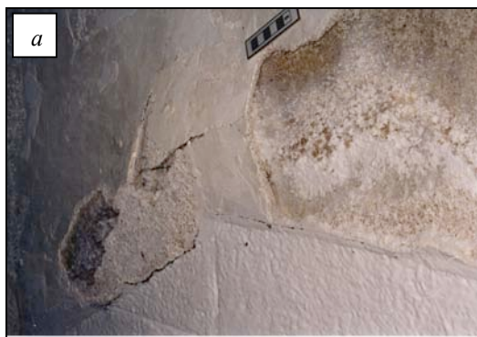
Figure 31: (a) Deterioration and breakdown of render associated with well-developed sulphate salt efflorescence; (b) staining of walls in the upper section of St. Peter's Tower caused by a combination of mould growth and corrosion from the service room above associated with moisture ingress from historic flooding of the lantern gallery.
