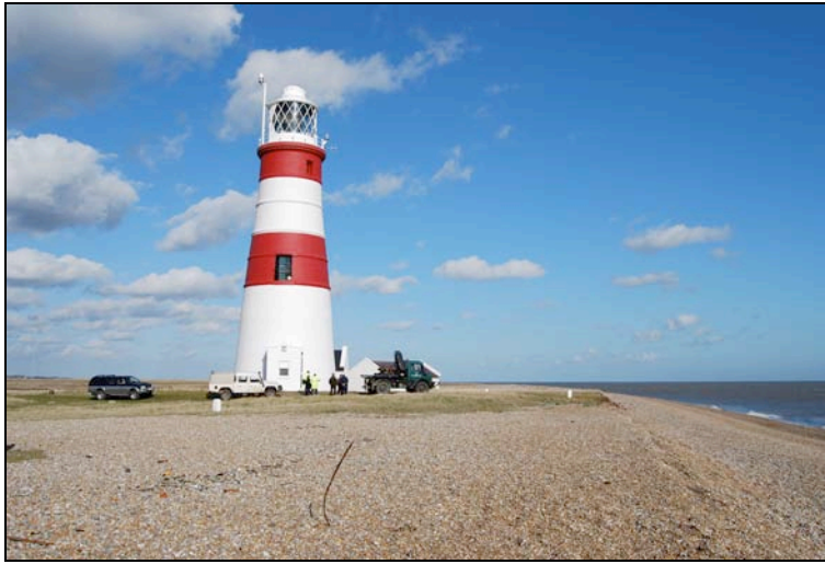
Figure 7: Orfordness Lighthouse located on a shingle spit which is undergoing significant coastal erosion that will eventually jeopardise the structural stability of the tower.
