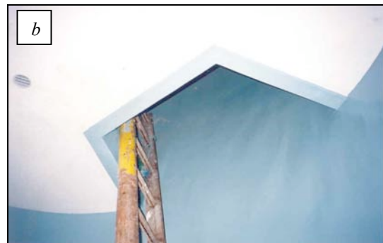
Figure 20: (a) Installation of ‘Delta Membrane System’ to stripped walls before plastering; (b) view of floor hatch after plastering and painting and before installation of new stairs.
