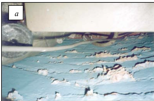
Figure 22: (a) Well-developed salt efflorescence associated with mortar lines on internal walls illustrating the effect of long-term salt-rich moisture ingress and chemical interaction with components of the mortar to form complex sulphate salts; (b) salt efflorescence has contributed to deterioration of painted surface of internal walls.
