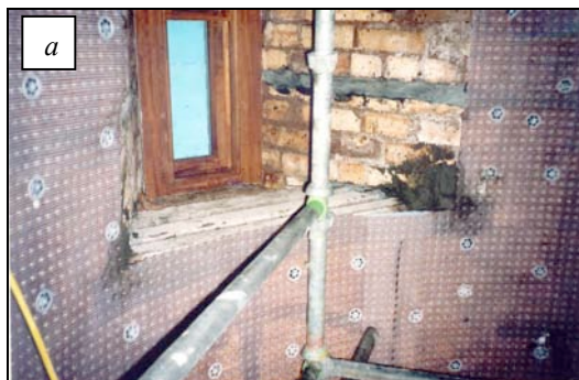
Figure 20: (a) Installation of ‘Delta Membrane System’ to stripped walls before plastering; (b) view of floor hatch after plastering and painting and before installation of new stairs.
