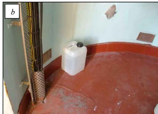
Figure 28: (a) Image showing corroded corner beading, flaking floor paint and corrosion related staining on walls; (b) example of flaking paint and bossed plaster.
