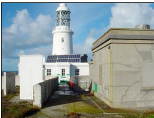
Figure 8: An example of different categories of condition with the operational lighthouse painted while the non-operational redundant engine room in the foreground is left unpainted (Round Island – TH site 31 in Figure 9).
