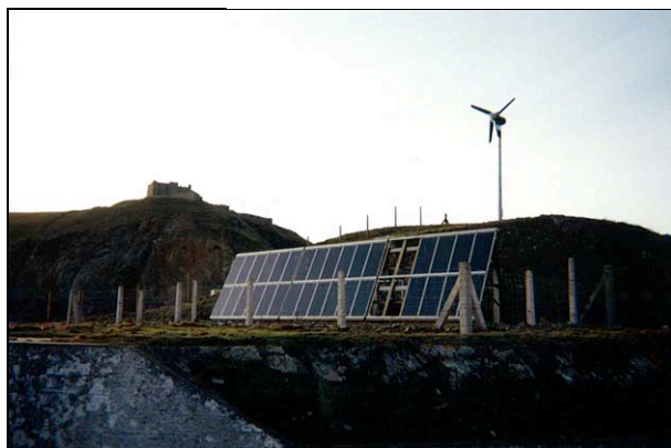
Figure 10b: Combination of a solar array and a Proven WT2500 wind turbine at Lundy South.
