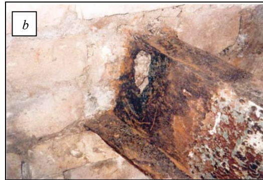
Figure 19: (a) View of ‘Wearite’ dry-lining and steel beams and timber floor joists; (b) severely corroded steel beam end behind the ‘Wearite’.
