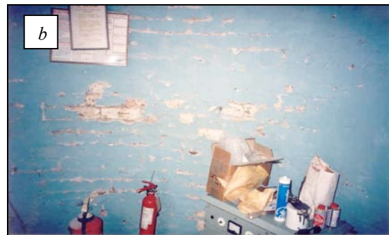
Figure 22: (a) Well-developed salt efflorescence associated with mortar lines on internal walls illustrating the effect of long-term salt-rich moisture ingress and chemical interaction with components of the mortar to form complex sulphate salts; (b) salt efflorescence has contributed to deterioration of painted surface of internal walls.
