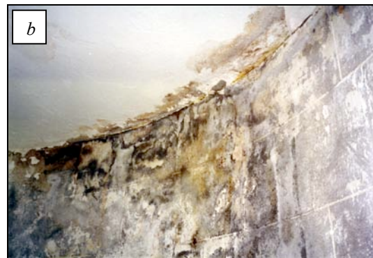
Figure 31: (a) Deterioration and breakdown of render associated with well-developed sulphate salt efflorescence; (b) staining of walls in the upper section of St. Peter's Tower caused by a combination of mould growth and corrosion from the service room above associated with moisture ingress from historic flooding of the lantern gallery.
