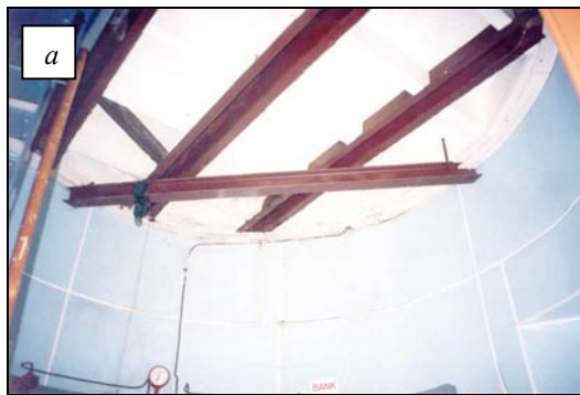
Figure 19: (a) View of ‘Wearite’ dry-lining and steel beams and timber floor joists; (b) severely corroded steel beam end behind the ‘Wearite’.
