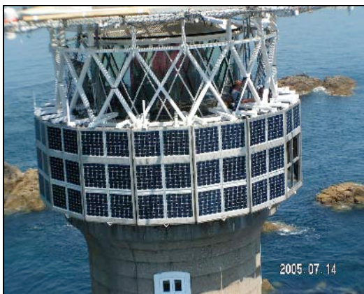
Figure 14: Longships lighthouse with solar panels to provide power to the navigational aid, main, standby and facilities battery bank. Brackets fitted for four 400W wind generators to supplement the charging regimes.
